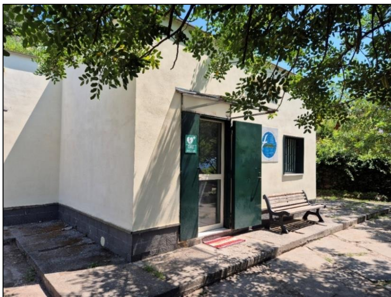
Figure 8: Service building promoting the cultural maintenance of the Monte Nuovo volcanic crater, own photo
